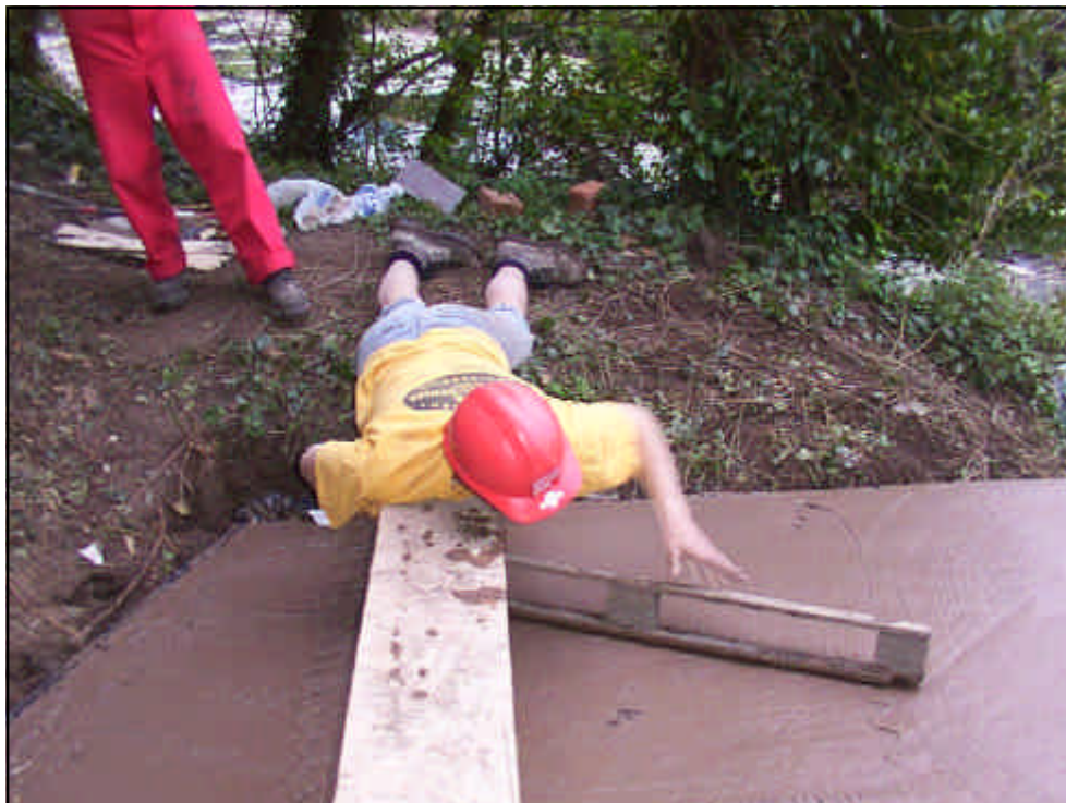
Matt putting the finishing touches on the concrete cap (Ed Walker)
