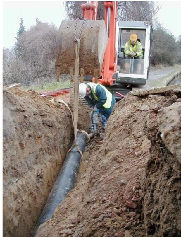
Tim removing concrete allowing final pipe placement (Helen Dobbie)
