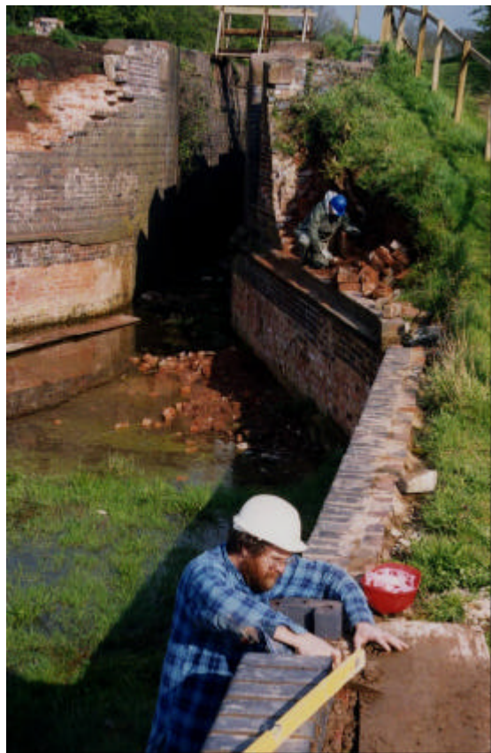
Martin laying bullnoses. (Droitwich Junction Canal, Tim Lewis)
